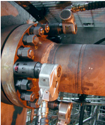
REACTOR-INLET FLANGE A,B,C (12) 1-3/8" B16 BOLTS
