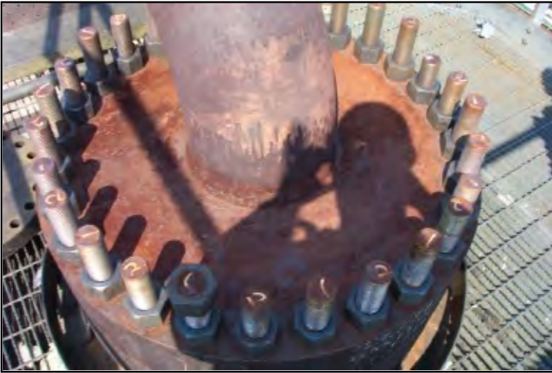
REACTOR 7V 108 (38) 1-7/8" B16 BOLTS
