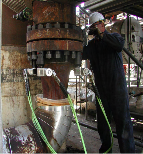
REACTOR-ELBOW FLANGE (20) 1-1/2" B16 BOLTS
