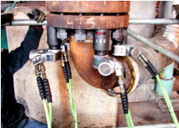
REACTOR-INLET FLANGE A,B,C (12) 1-3/8" B16 BOLTS
